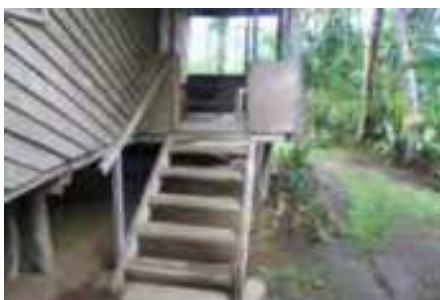
✓ Very good steps, well spaced, good bottom landing stone, just needs an outer handrail!
