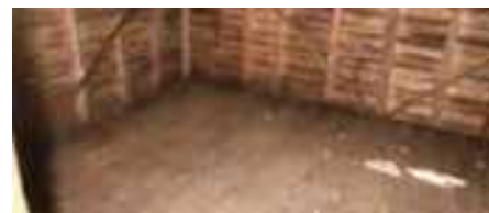
✓ Timber external cladding. Timber floor, nails need to be punched or they may puncture trekker's inflatable mattresses.
