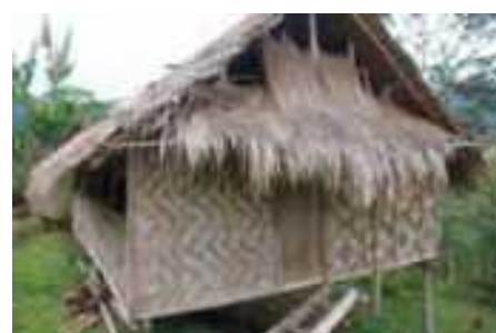
✗ Steps do not have a landing and do not match the door.
