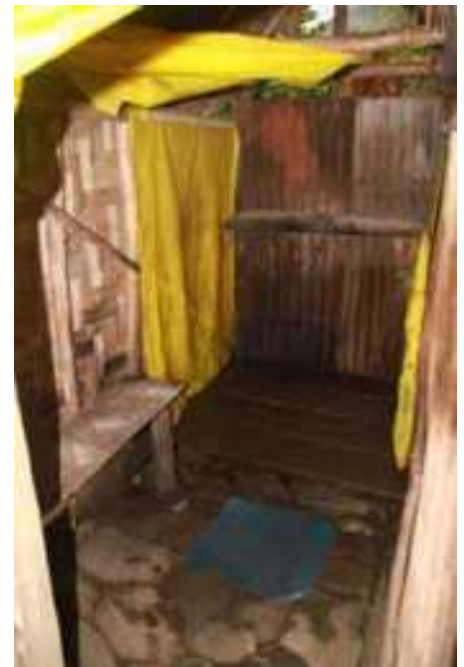
✓ Looking inside, seat to put towel, clothes and change. Well drained rocks in outer area and timber grate on shower floor. Inner shower curtain. Soap/shampoo shelf.
