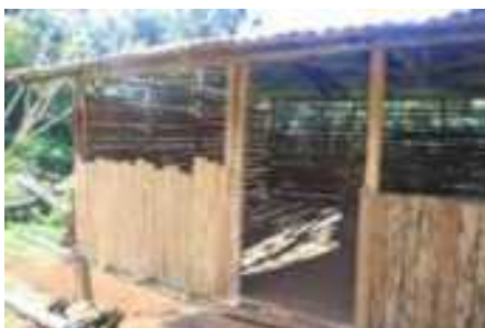
✓ Different wall cladding, split timber and saplings.
