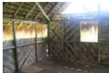
✓ Split bamboo wall cladding, appear durable and longer lasting.
