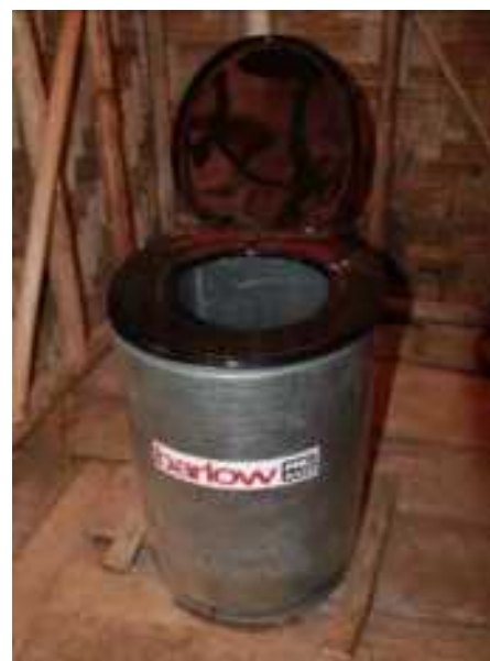
✓ Barlow galvanised iron pedestal and plastic seat.
